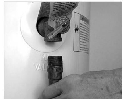
Figure 20. Removing the T&P Relief Valve discharge pipe.
