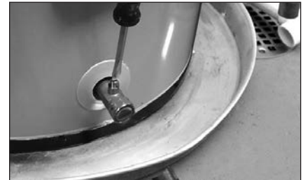
Figure 19. Draining the old water heater.
