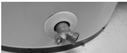
Figure 8 - Drain Valve
