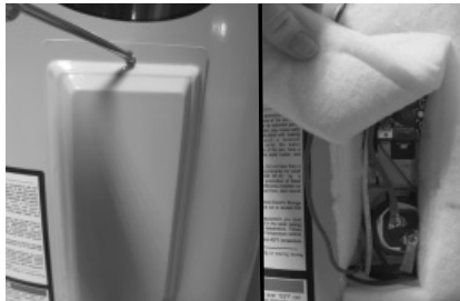
Figure 12 - Element Access Panel/ECO Compartment
